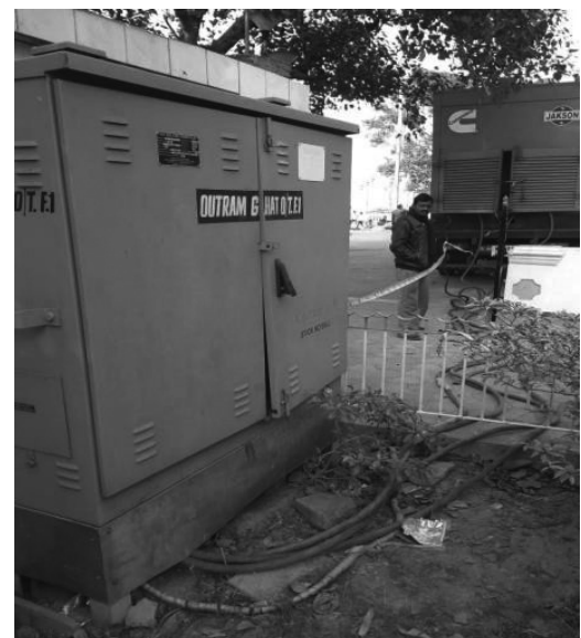
Photo No. 18: Emergency supply with mobile generator
