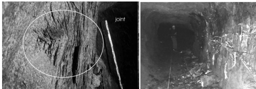
Figure 2: Examples of spalling
