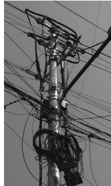
Photo No. 8: OH pole crowded with network of Cable TV
