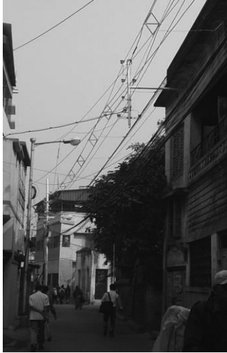
Photo No. 12: OH system with diamond type spacers
