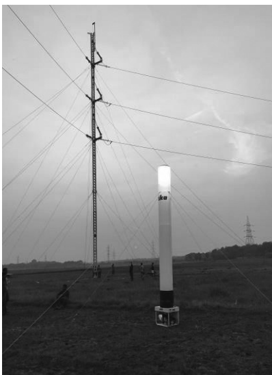
Photo No. 38: ERS tower under erection
