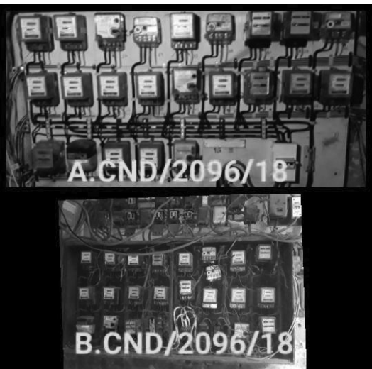
Photo No. 34: Meter board before and after renovation in public place
