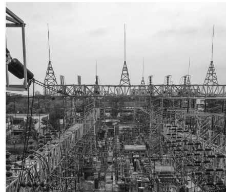
Photo No. 31: Outdoor yard with DSLP
