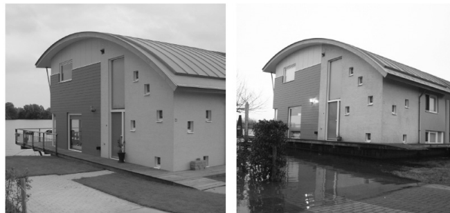
Figure 7: Amphibious house of Maasbommel, the Netherlands, before and during flood
