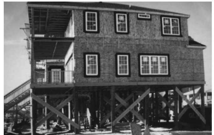
Figure 9: Foundation bracing
