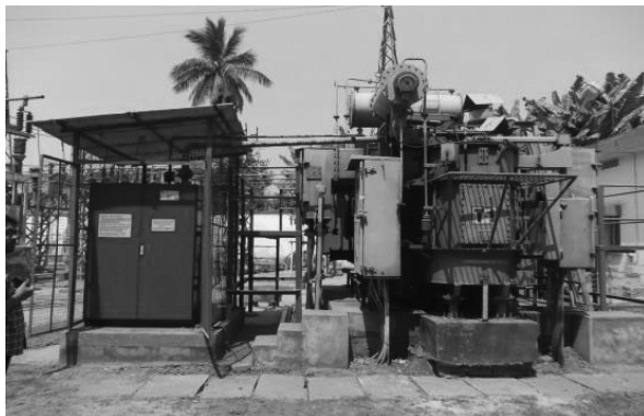
Photo No. 16: NIDS protection of power transformer
