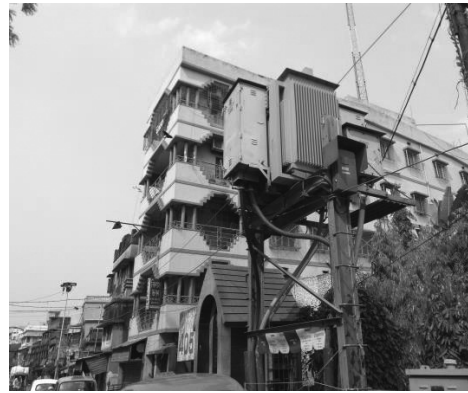
Photo No. 14: Dry type Dist. Trf. in congested place
