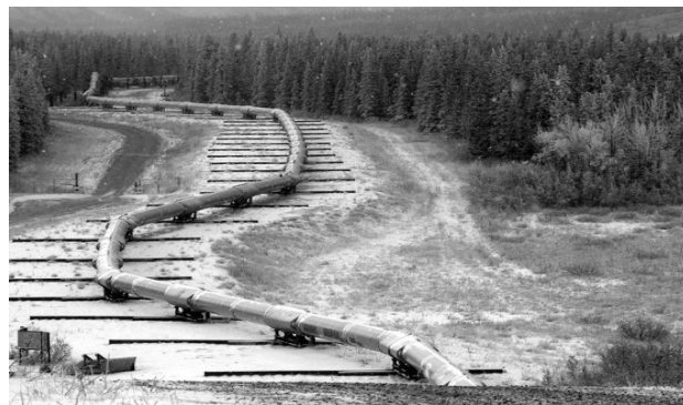
Figure 55: Zig Zag pipe line led in Alaska which is crossing the Fault line
