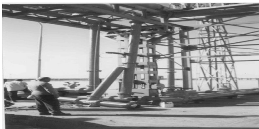
Figure 4: Two fire water lines on the IFFCO jetty experienced failure near the elbow, as well as near the flange on the vertical branch.(7.6M, January 26, 2001, 50 km epicentral distance, 0.37 g PGA estimated)
