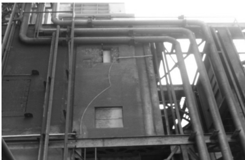
Figure 41: BACW piping continue at KLTPS (No damage)(Bhuj earthquake, 7.6 M, 2001, 0.22g pga)
