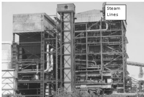
Figure 37: Steam line coming down from the boiler drum. (No damage) (Bhuj earthquake, 7.6 M, 2001, 0.24g pga)
