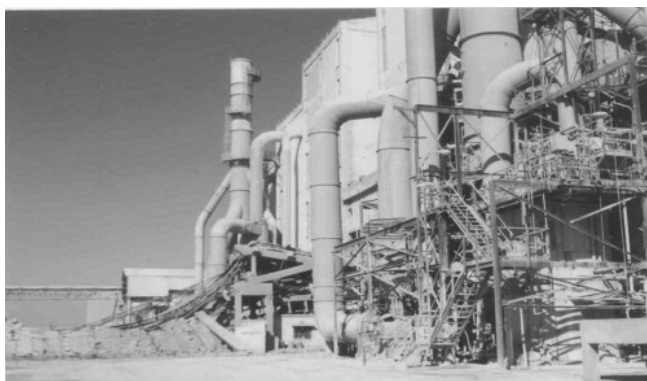
Figure 57: Damage to the piping due to falling of conveyor gallery on the pipelines at IFFCO plant which witnessed 7.6 M earthquake of 26 Jan 2001., 0.37 g Pga
