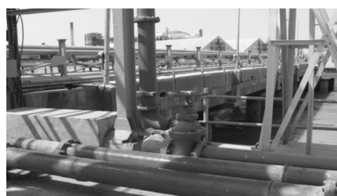
Figure 7: Third flexible line coming down from the structure (No damage)(7.6M, January 26, 2001, 50 km epicentral distance, 0.37 g PGA estimated)
