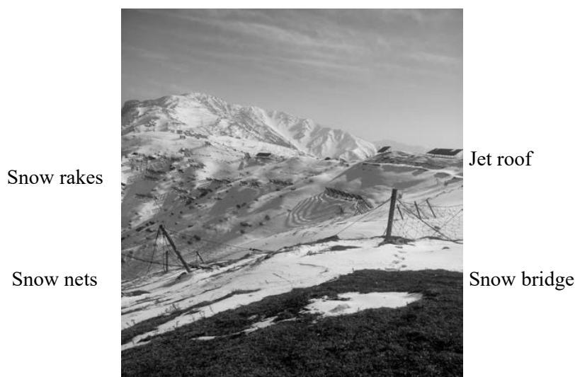
Figure 10: Supporting structures installed at avalanche site D-10 (Jammu and Kashmir)
