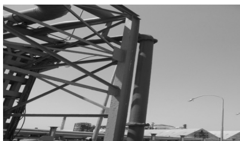
Figure 6: Third flexible lines coming down from the structure. (No damage)(7.6M, January 26, 2001, 50 km epicentral distance, 0.37 g PGA estimated)
