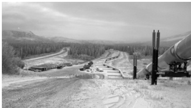
Figure 54: Zig Zag pipe line led in Alaska which is crossing the Fault line
