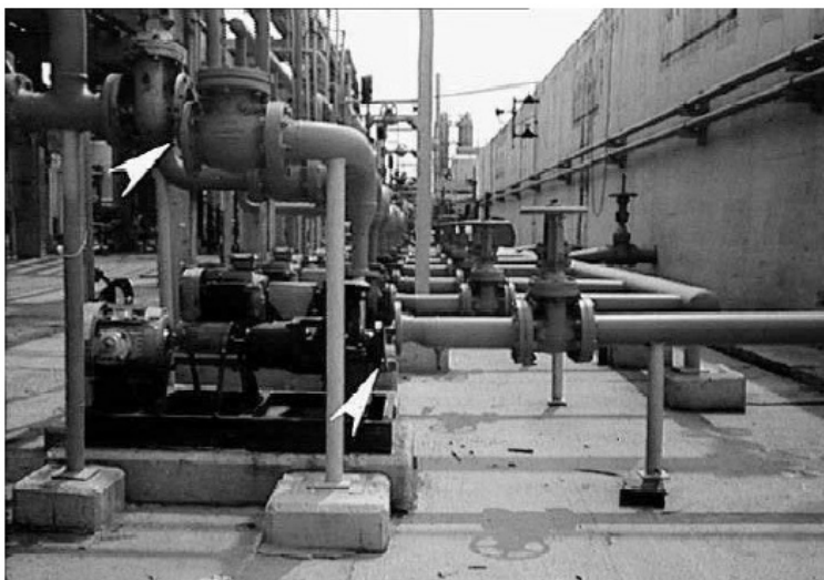
Figure 50: Seismic ground settlement
