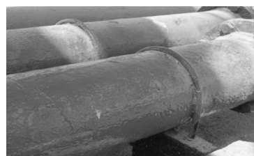
Figure 15: Close view of U-clamp support on fire water on main jetty(No damage)(7.6M, 26th Jan 2001, 50 km epicentral distance, 0.37 g PGA estimated)
