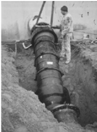
Figure 30: Flexible connection being provided at the tank outlet
