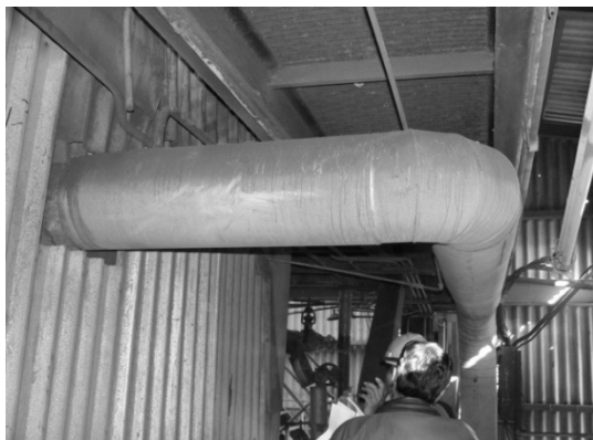
Figure 18: Vent line connected to the Economiser line which saw failure at the elbow due to large seismic inertia load from the steam drum (7.6M, January 26, 2001, 40 km from the fault plane, 0.22g)
