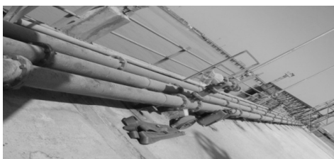
Figure 14: Fire water on main jetty(No damage)(7.6M, 26th Jan 2001, 50 km epicentral distance, 0.37 g PGA estimated)
