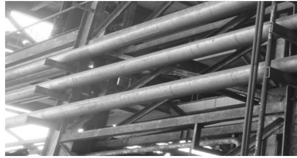
Figure 40: BACW piping at KLTPS (No damage) (Bhuj earthquake, 7.6 M, 2001, 0.22 g pga)
