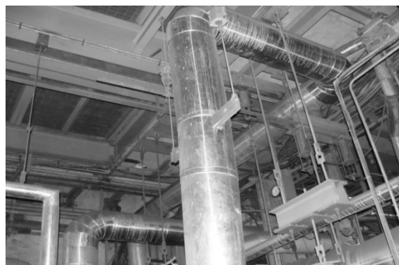
Figure 38: Spring support for steam piping at GEB, Sikka (no damage) (Bhuj earthquake, 7.6 M, 2001, 0.24g pga)
