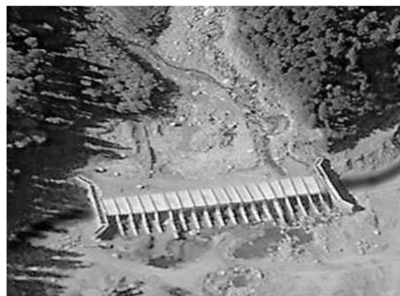
Figure 7: Snow Gallery constructed at MSP-7 (Manali, Himachal Pradesh, India)
