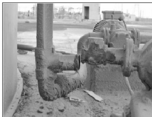
Figure 25: Failure of Rigid Piping during Bam earthquake (Iran) (M=6.5, ED=5 km, 27 Dec, 2003) (Damage)
