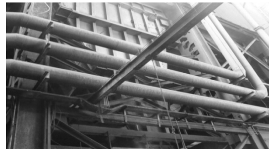
Figure 42: Dead weight support scheme in BACW and TACW line (No damage) (Bhuj earthquake, 7.6 M, 2001, 0.22g pga)
