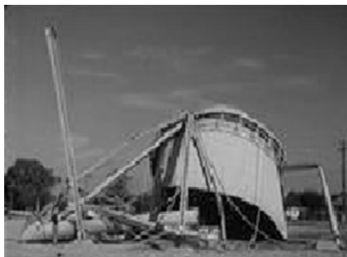
Figure 26: Elevated tank collapsed, kern country earthquake california, 1952, M 7.5, (Damage)
