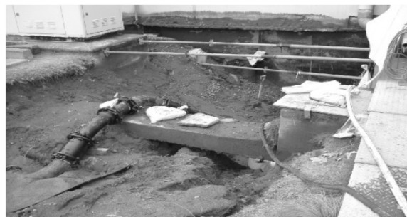
Figure 45: Failure of a buried piping in Kashiwazaki Kariwa NPP which experienced 6.8 M earthquake at 16 km epicentral distance & 0.68g PGA
