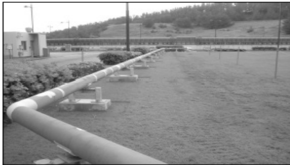
placing fire piping above ground
