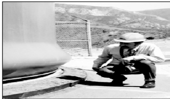
Figure 27: Elephant foot bulging of a tank wall, 1971 san fernando earthquake, M=6.6 , ECD=10 km, H/D=0.714 (Damage)
