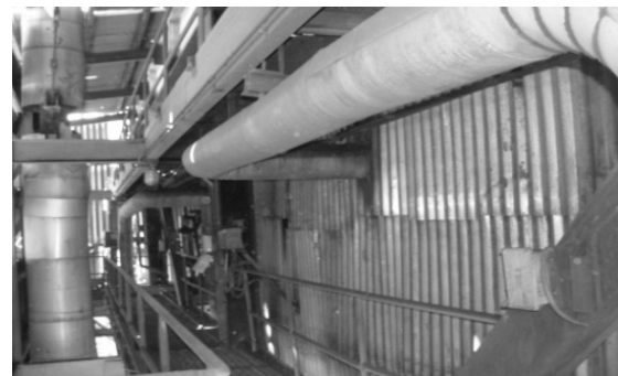
Figure 17: The two economiser lines to the steam generator. The vent lines are connected to each of the economiser lines which are not visible in the picture (No damage to the economiser lines)(7.6M, 26 th Jan 2001, 40 km from the fault plane, 0.22g)
