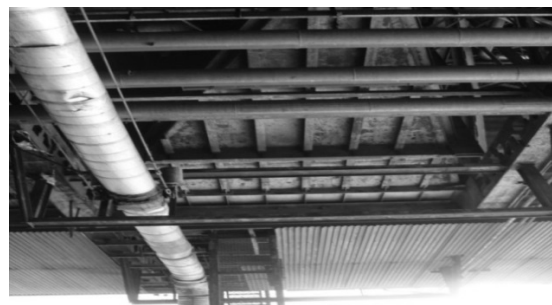
Figure 36: Supporting arrangement in Vertical steam line of Sikka thermal power plant (GSECL), Jamnagar (No damage) (Bhuj earthquake, 7.6 M, 2001, 0.24g pga)
