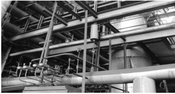
Figure 39: Feed water header at 13m Elevation. (No damage) (Bhuj earthquake, 7.6 M, 2001, 0.24g pga)
