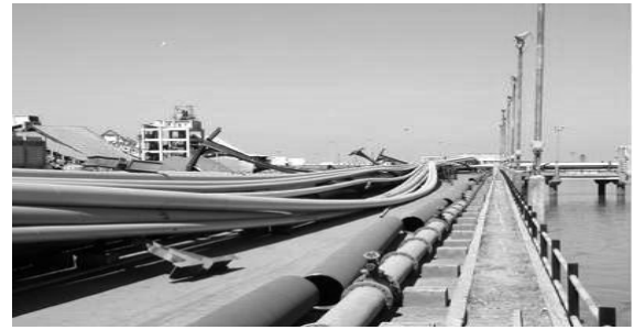
Figure 32: Damage to the pipe racks and pipelines falling on the KPT jetty (7.6M, January 26, 2001, 50 km epicentral distance, 0.37 g PGA)
