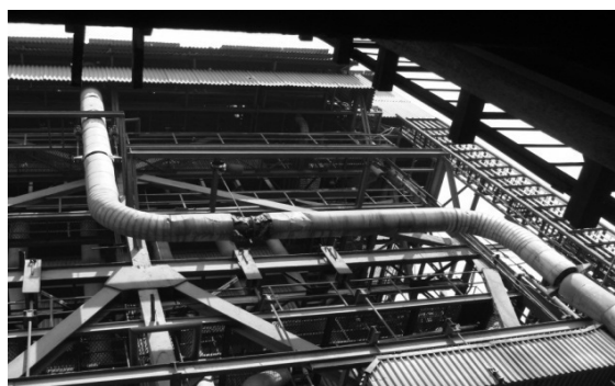
Figure 35: Steam line coming down from the boiler drum. (No damage). The steam line at Sikka thermal power plant (GSECL), Jamnagar. If the piping spans are large and the fundamental frequency less than 0.1 Hz, the piping may see large displacement and may swing and impact with adjacent pipe or equipment or structure. Such long spans of 20 m should be provided with cable bracings. (Bhuj earthquake, 7.6 M, 2001, 0.24g pga)
